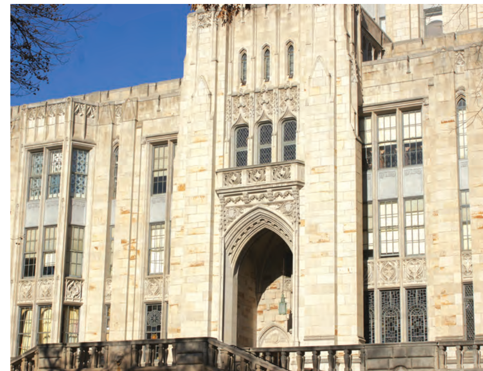
Cathy, as the tower is affectionately known, has several grand entrances, including this imposing one on the west face, along Bigelow Boulevard.
